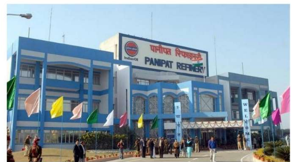
IOCL Panipat Refinery
